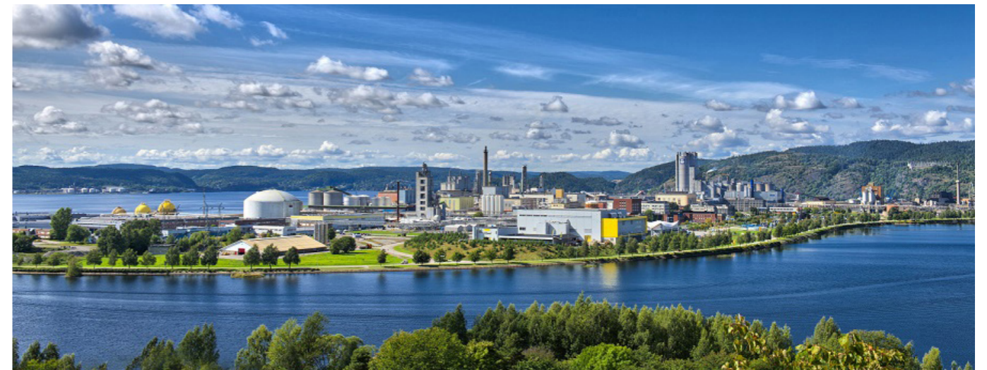
Herøya Industripark AS, Porsgrunn. Foto: Tom Riis/Herøya Industripark AS
